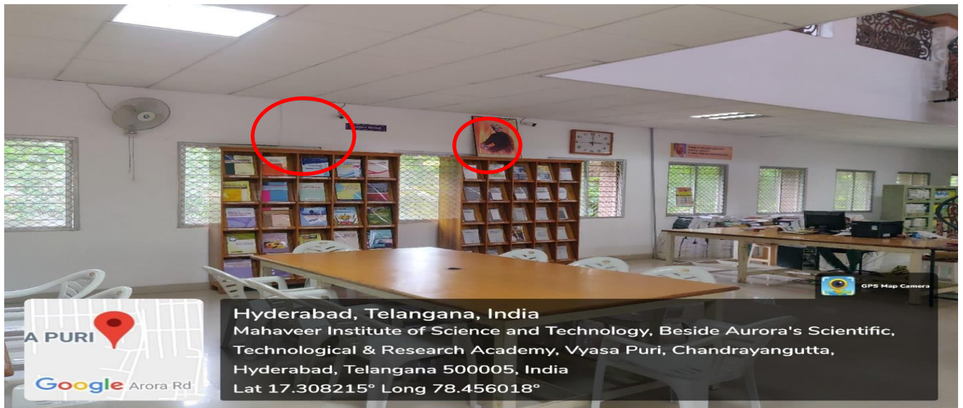
vii. Camera Installed in the Library
